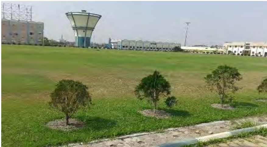
WTP land owned by HIDCO (with existing WTP operated and maintained by PHED)
