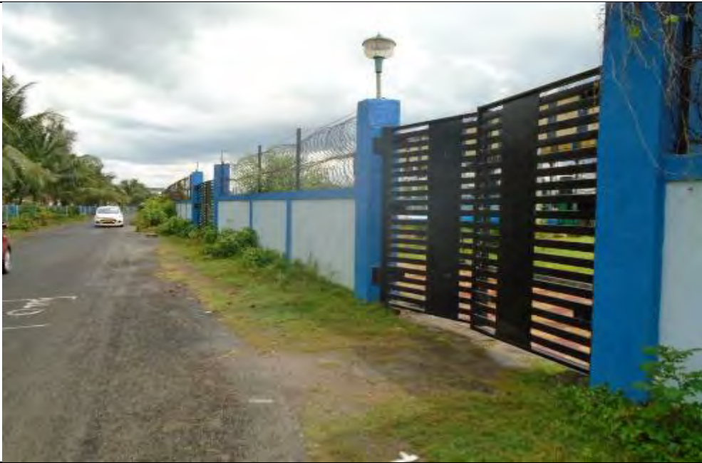
End of Transmission Line at BS-1
