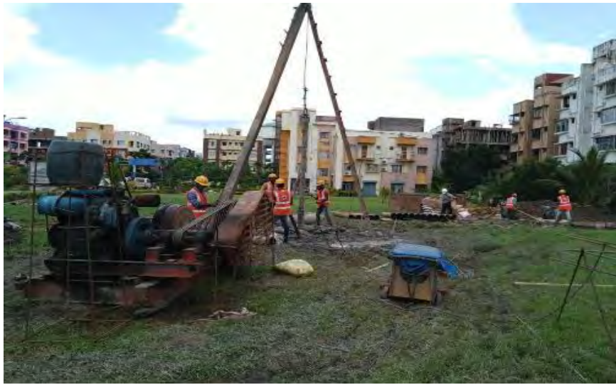
Work at going on WTP Site
